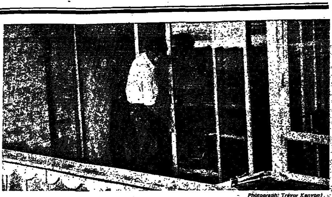
Double glazing in Sussex. Alcan installers Dave and Martin fit Alcan's aluminium-framed double-glazed sliding patio doors in place of the old rusted windows taken out of a third-floor balcony room. The door and windows on the right have still to be replaced. Enquiries Peter Newman, Regional Sales Manager, Alcan Design Centre, 5 Portmore Park Road, Weybridge, Surrey.
